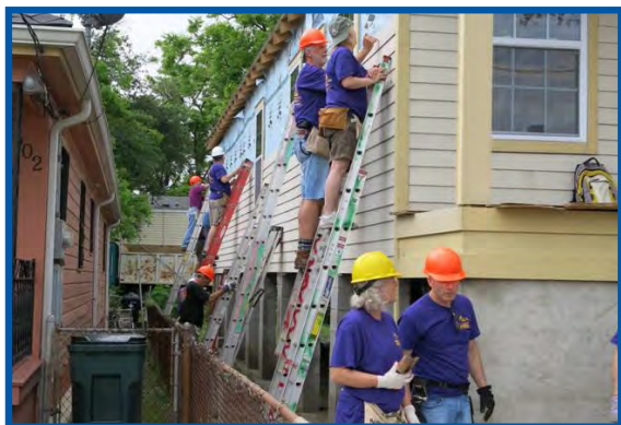
Installing siding.
