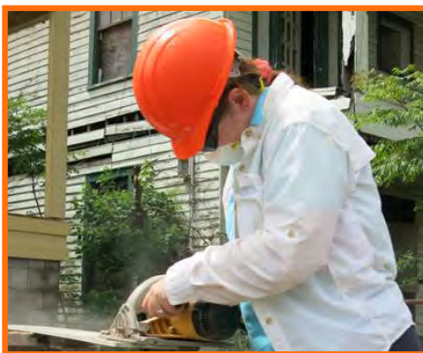
Cutting some siding.
